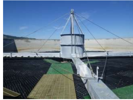
New rotary distributor, Biotower 2
