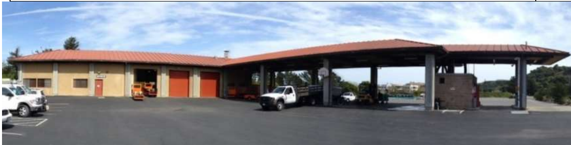
Maintenance Building: Standing seam metal roof
