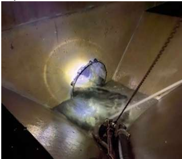
48" Primary Effluent Pipe – Interior
