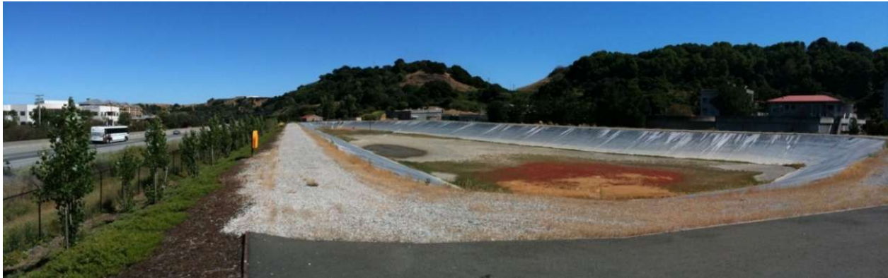
Effluent Storage Pond
